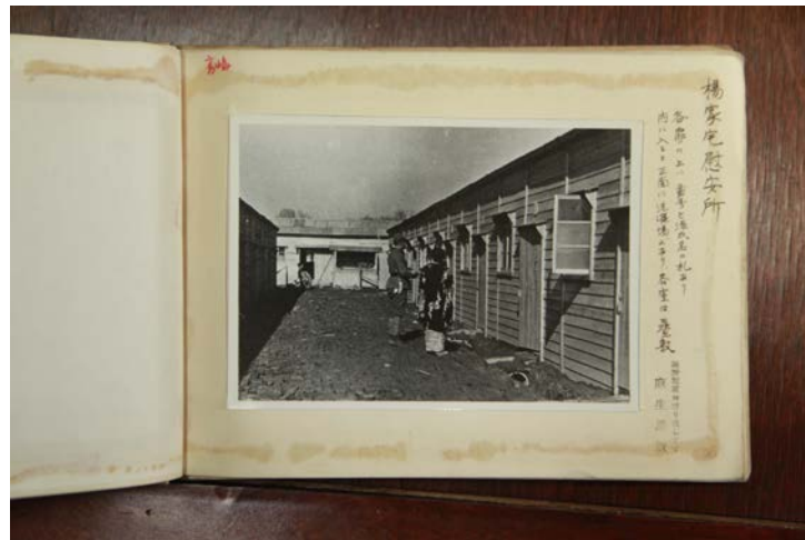
Figure 1. The photograph the my father left in the album says “Yang Jia Zhai Comfort Station. Above the doors to each room, there is a tag with the family name written on it. Inside, there is a bath, and each room is tiled with tatami mattress”. When he was alive, my father denied allegations that the Comfort Women were “sex slaves”.
